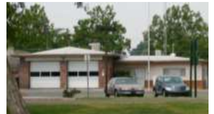
Rio Linda Fire Station showing original brickwork
