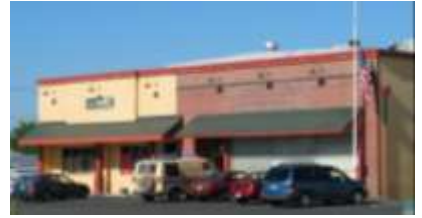
These simple commercial buildings have been articulated with variations in color and materials and the use of awnings and a roof cornice.
