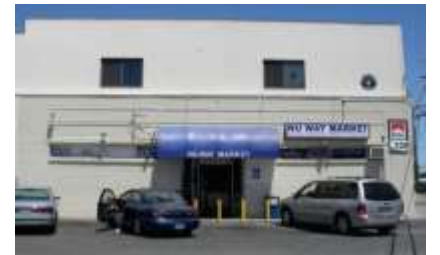
The Nu Way Market includes brick and concrete masonry on the ground floor with wood siding on the second story. The large surface planes of the building should be articulated through the use of color and contrasting use of the two materials.
