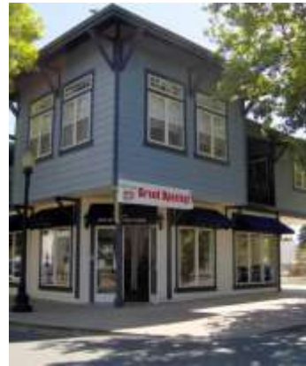
Corner buildings should be two-story and with vertical elements that reinforce the building's gateway location.
