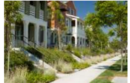
Infill construction such as these townhomes should front onto M Street with entries at or near the build-to line at the back of the sidewalk.
